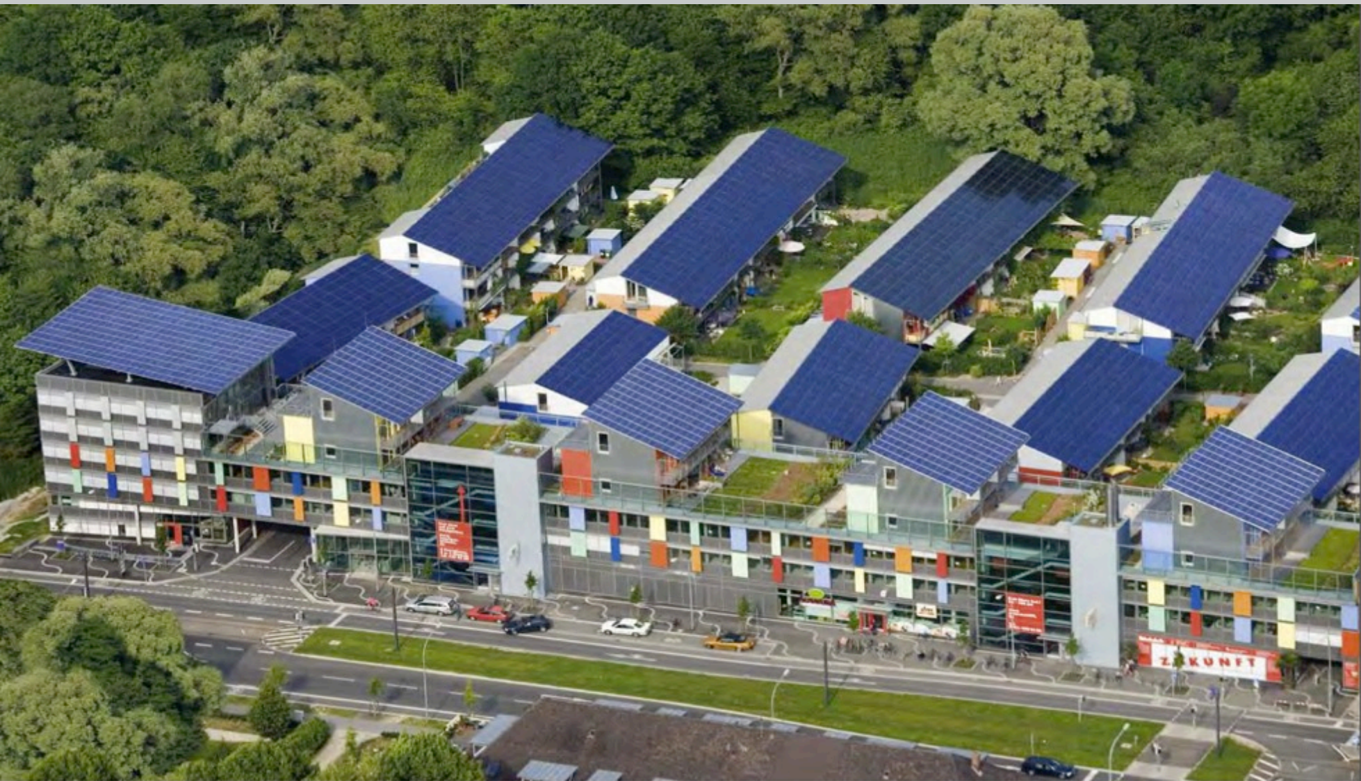
Caption: Plus energy houses are designed to produce more energy than they consume in the course of the year.
