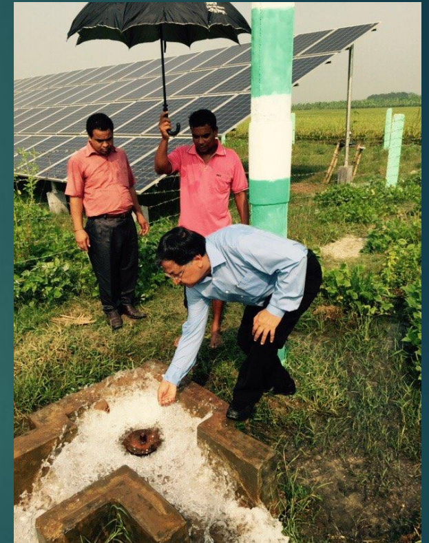
Water Discharge by a Solar Irrigation Pump installed in Kustia by BGEF
