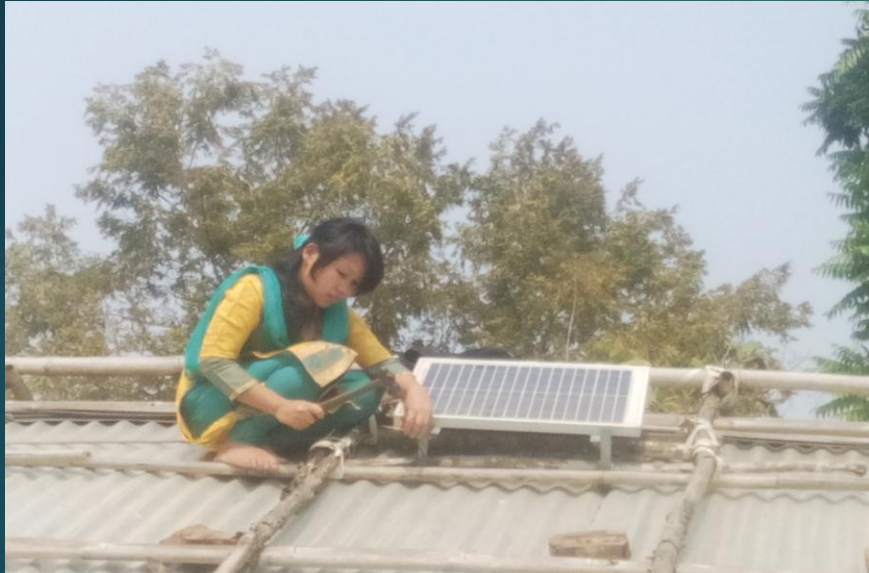
Solar Home System (SHS) installation
