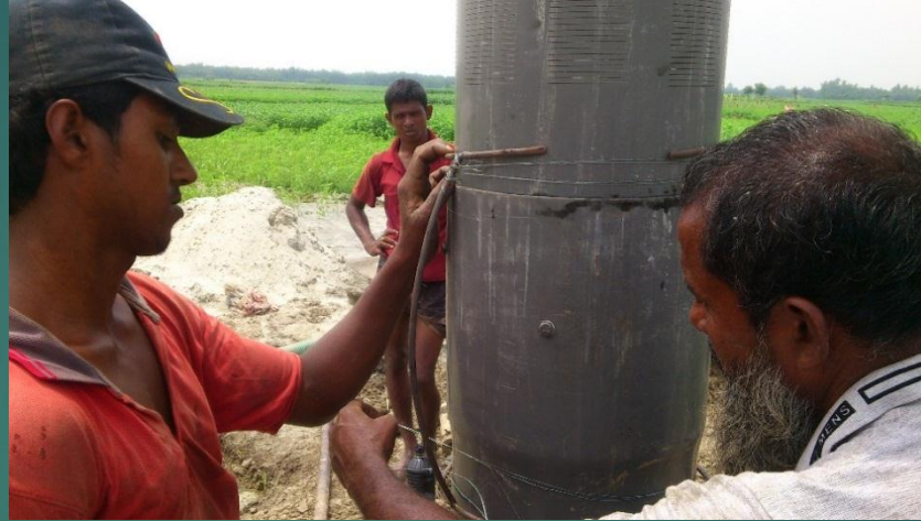
Pipe boring process
