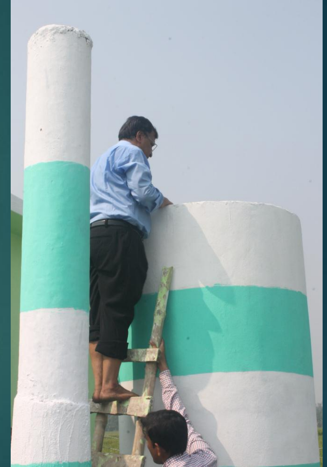
Inspecting water reservoir tank
